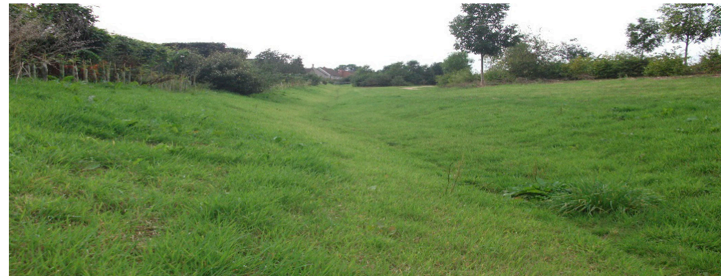
Example of SuDS swale: Long Ashton
